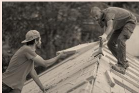
A. Soft wood fibre pieces are placed from ridge to eaves to avoid sliding on top of them while fixing.
