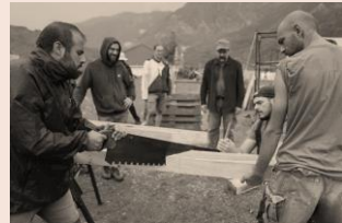
Cutting wood using a 2-person traditional saw
