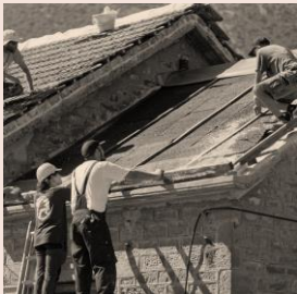
B. Boards of cork applied. Attention needed while placing to avoid cracks.
