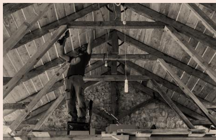
The new structure (hammer beam truss) after the modifications
