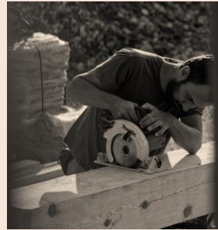
Forming notches using an electric circular saw
