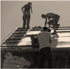
B. Layers of sheep wool between the battens. The wool is cut in slightly bigger pieces, in order to be tightly fixed.
