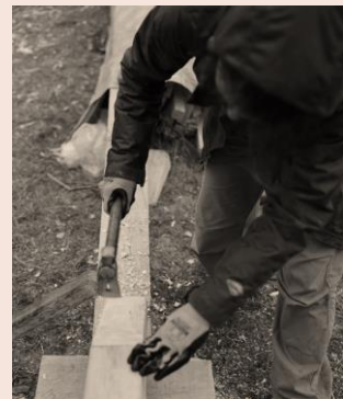
Forming wood connections of the roof trusses using an adze
