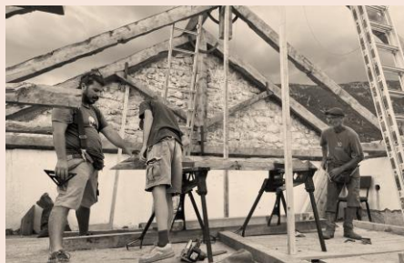
Modifications and cuts on the existing (old) trusses
