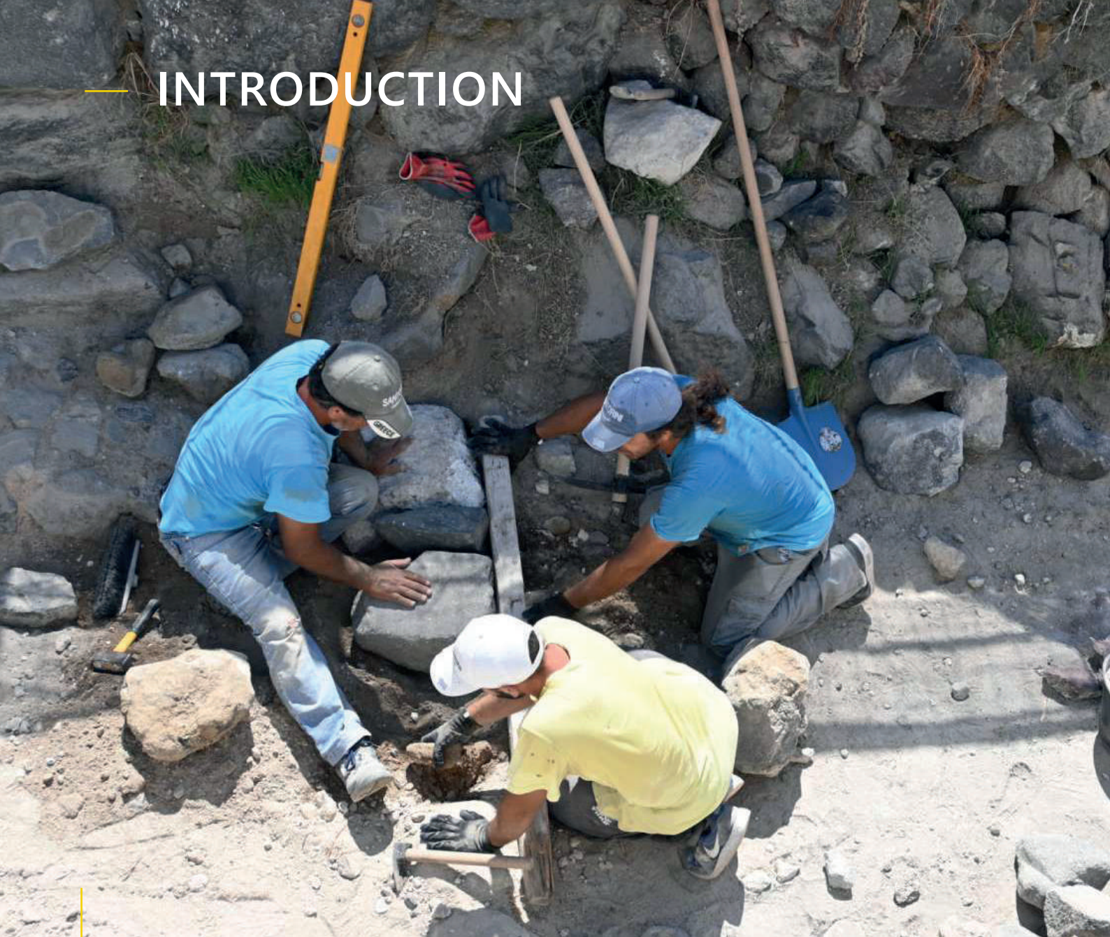
Trainer and apprentices while leveling the cobblestone during restoration works, Cyclades, Greece.
